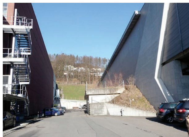
Rand A2 Portal Sonnenberg-tunnel
